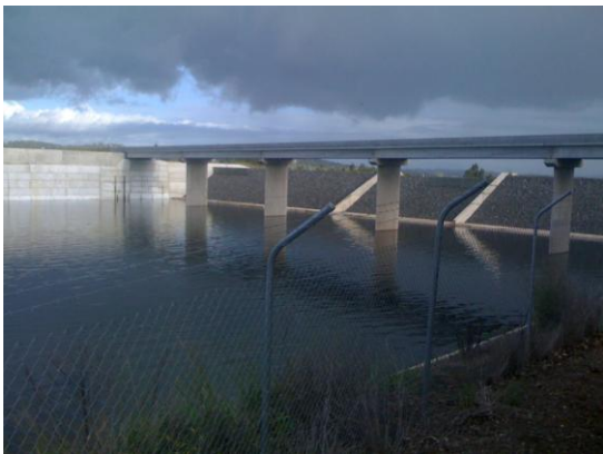
Wivenhoe Auxiliary Spillway
